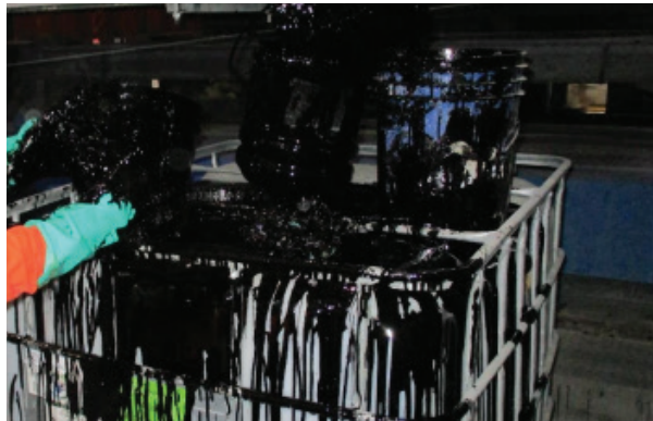
Housekeeping issues with asphaltic-based open gear lubricant
